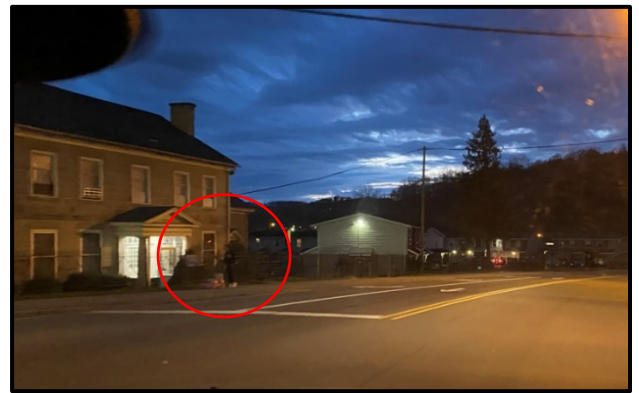
Photo 2: Inadequate Lighting Conditions at Intersection
