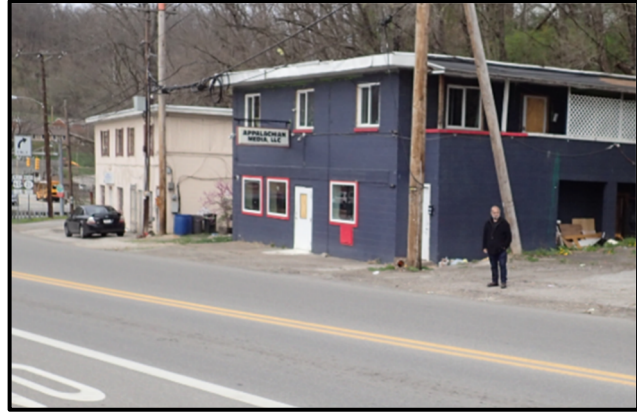
Photo 5: Buildings on Northern Side of Washington Street
