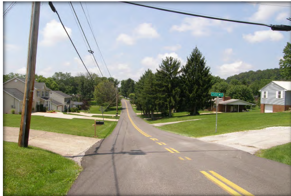
Figure 8: Looking West on Mount Vernon Road Showing Typical Utility Conflicts
