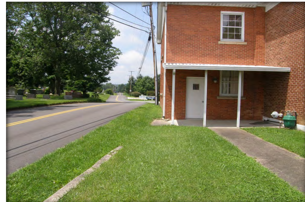
Figure 4: Mount Vernon Baptist Church Addition (Looking West)
