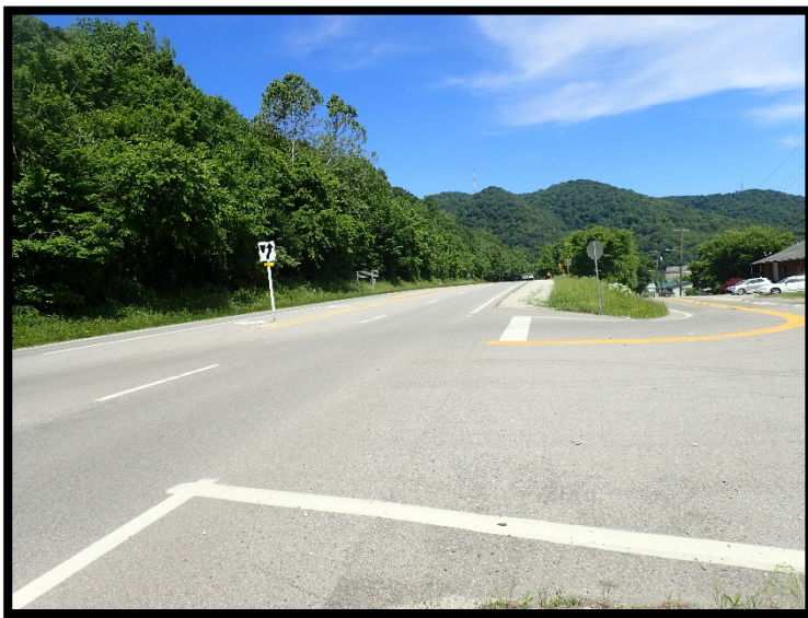
Photo 4: US 60 & Hull Ave Pavement
