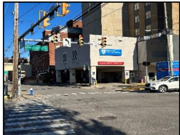
Photo 4: Sun Glare Affecting Signal Head Visibility at Washington Street and Brooks Street
