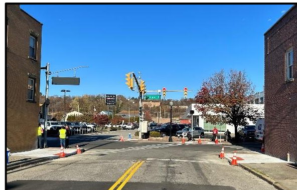
Photo 5: Offset Intersection at Bradford Street and Sun Glare Impacting Signal Head Visibility
