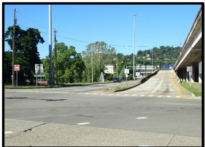
Photo 5: I-64 Ramp at Pennsylvania Ave North & Lee St
