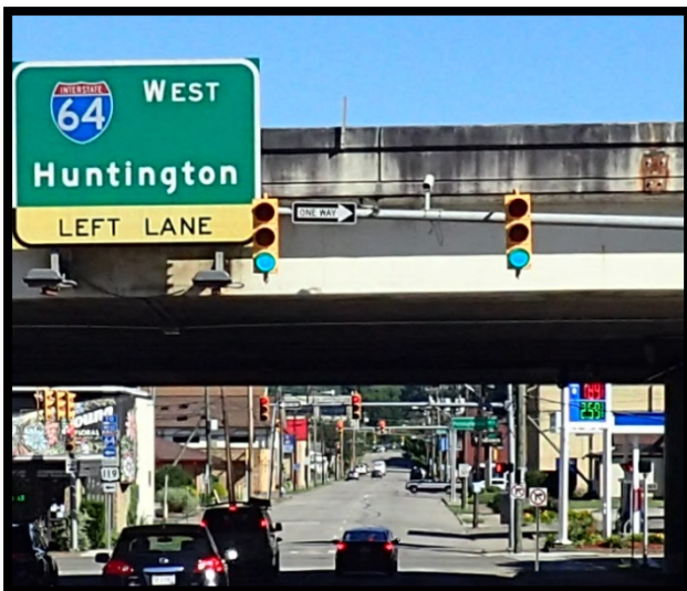
Photo 2: Signals Westbound on Randolph Street
