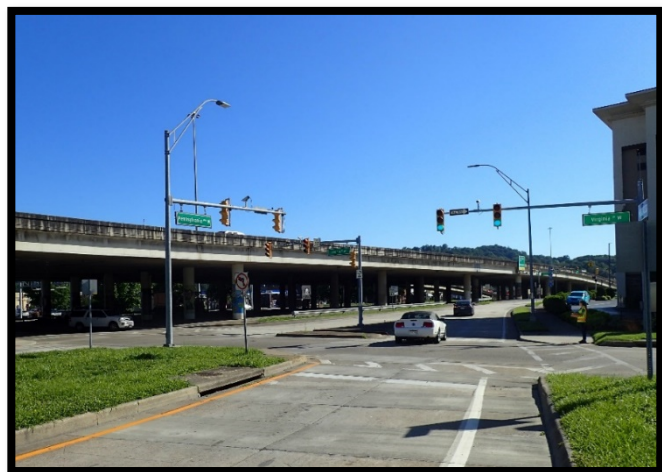
Photo 1: Pennsylvania Ave N and Virginia St W Off-Ramp Signal
