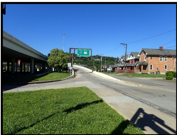
Photo 14: I-64 Ramp at Pennsylvania Ave S and Virginia St W
