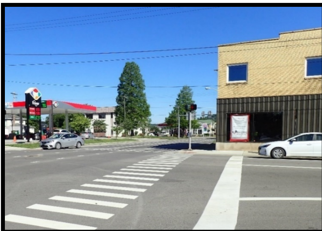
Photo 10: Building on Northwest Corner
