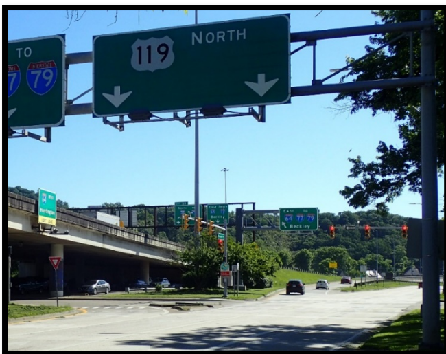
Photo 6: I-64 Ramp at Pennsylvania Ave N and Washington St
