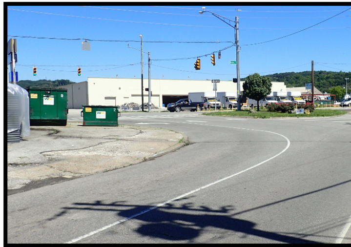
Photo 5: Patrick St and Kanawha Blvd W Westbound Approach
