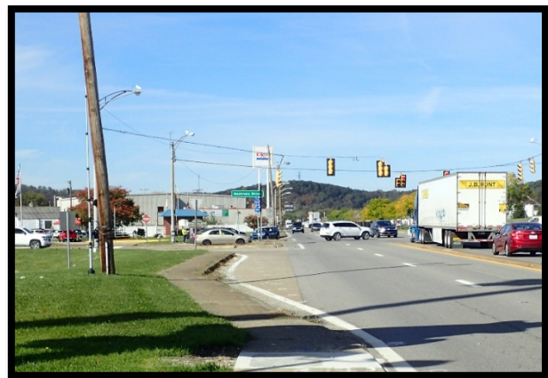
Photo 4: Acceleration Lane for Northbound Right-Turn
