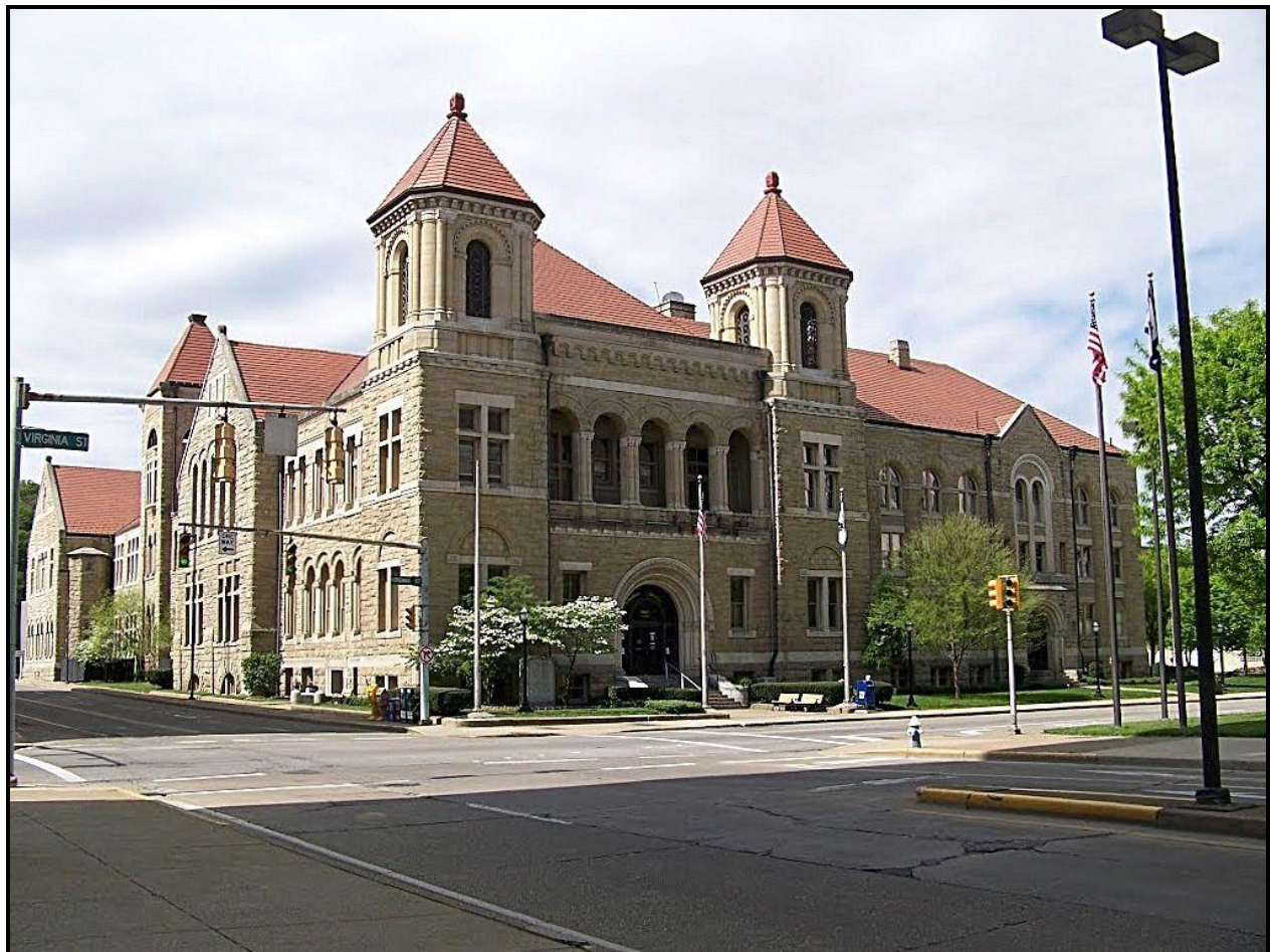
Kanawha County Courthouse
