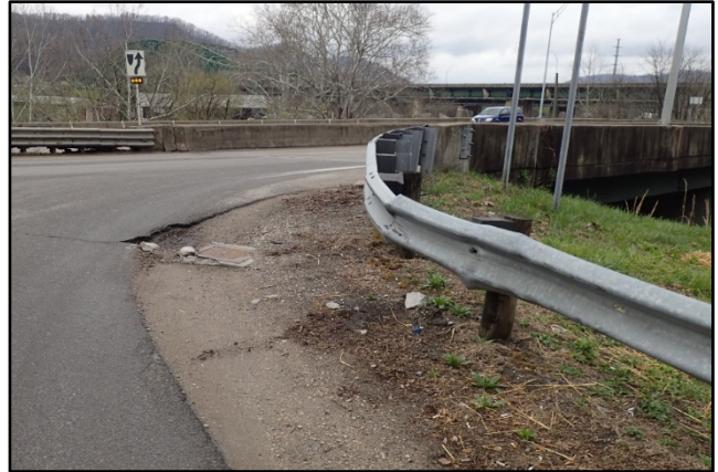
Photo 5: Guardrail on Northern Corner of Intersection
