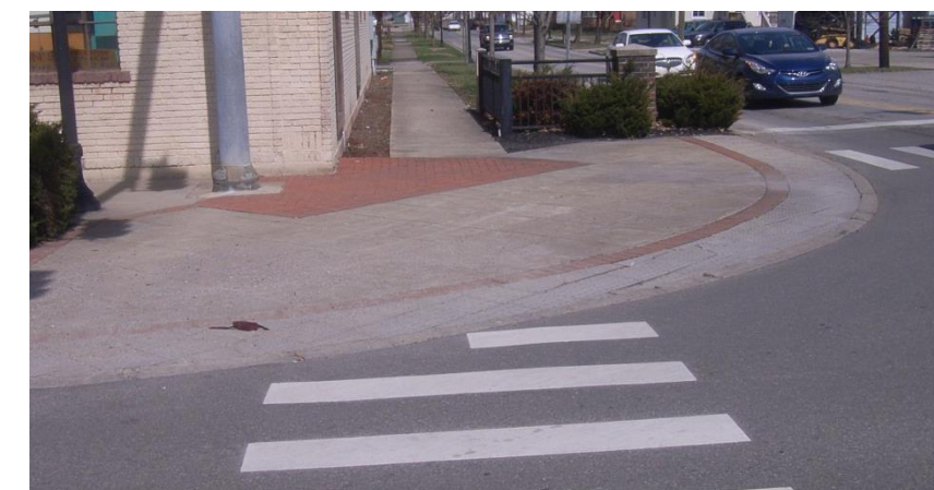
Figure 5-15: Curb Ramp at Third Street and Sixth Avenue
