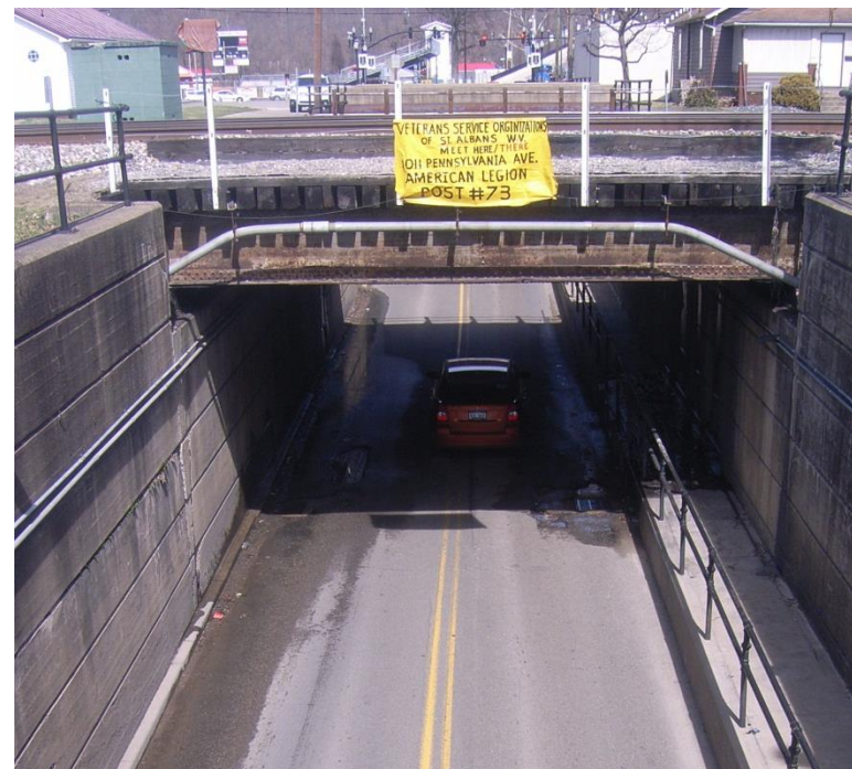
Figure 5-1: Third Street at CSX Underpass Looking North
