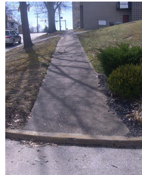
Figure 5-13: Steep Sidewalk at Main Street
