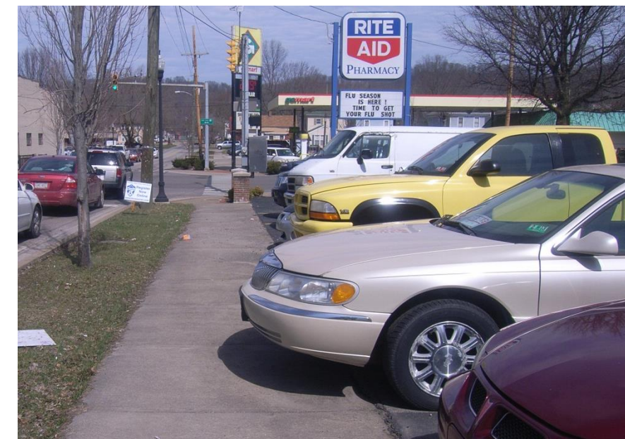
Figure 5-14: Parked Car Partially Blocking Sidewalk along Third Street near Sixth Avenue
