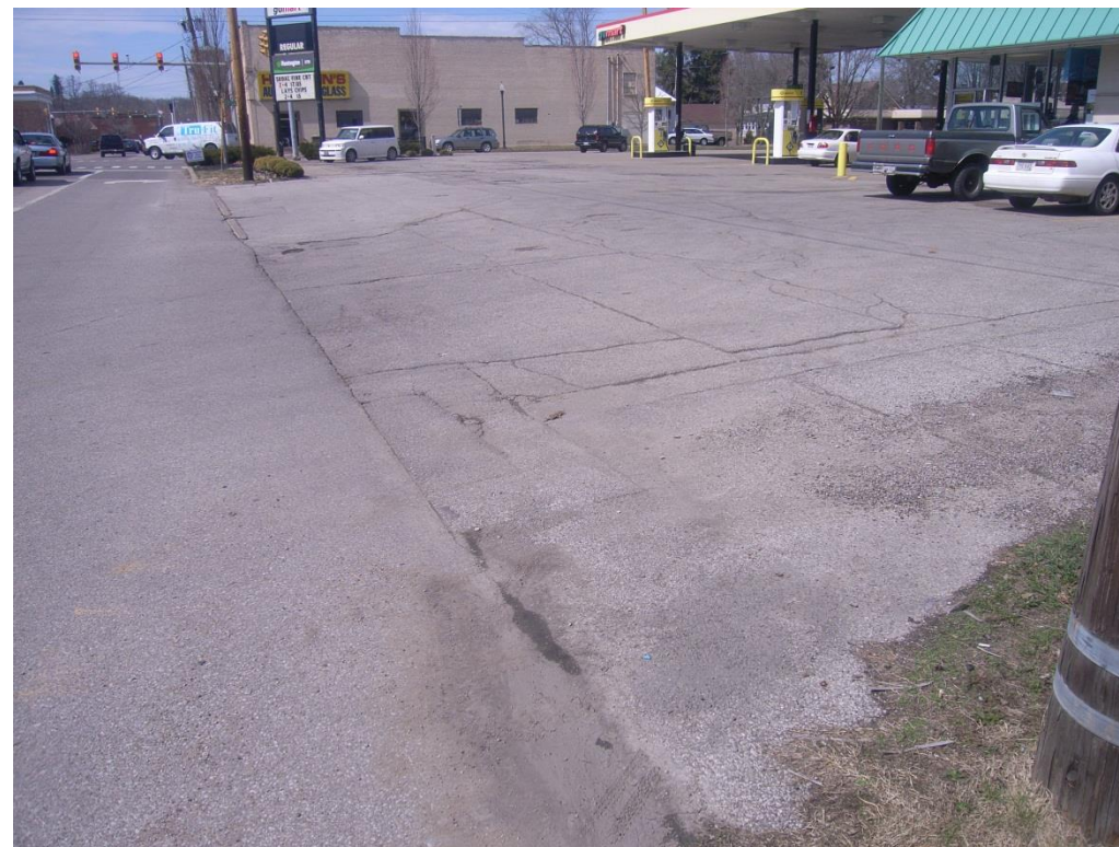
Figure 5-8: Go Mart Driveway along Sixth Avenue
