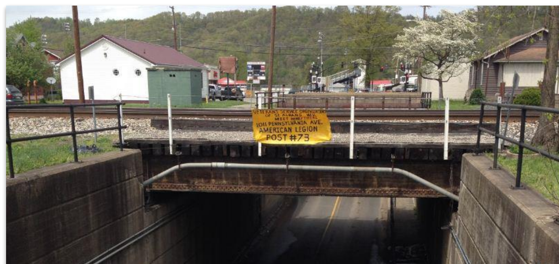
Figure 5-30: Third Street Underpass with CSX Corporation Railroad Bridge (Facing North)
