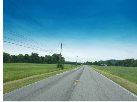
#10 WV 817 – Winfield to Hurricane Creek Road
