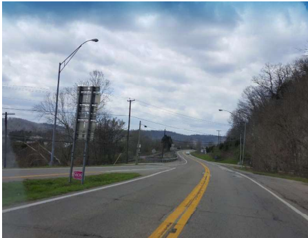
#1 WV 62 – Winfield Bridge to Eleanor
