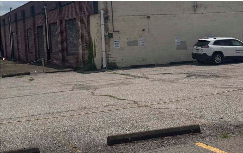
View looking east toward Segra.
