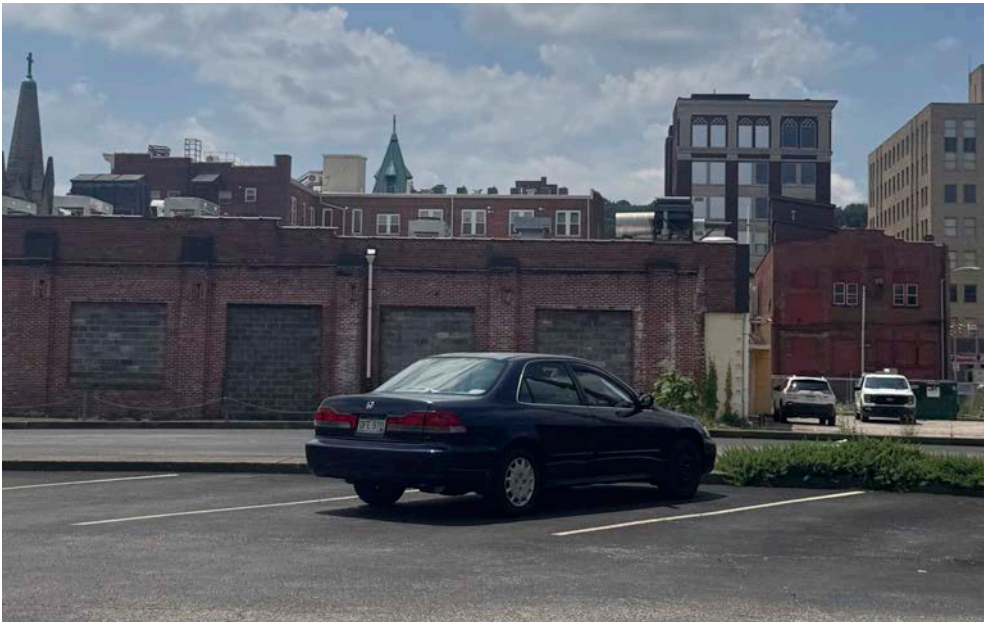
View looking south toward Segra and inside of Huntington Bank drive through lot.
